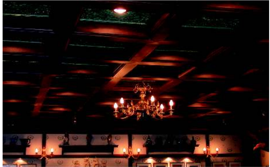
Ceiling Rafters with Phantom Veil
